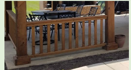
Post Base and Railing
