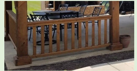
Post Base and Railing
